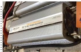
169A 10000 Watt 12 Volt Aims Power DC to AC Power inverter Installed in 2022
