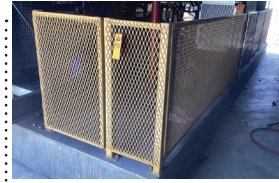
172 58' Safety Railing with Access gates
