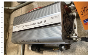
169D 10000 Watt 12 Volt Aims Power DC to AC Power inverter Installed in 2022
