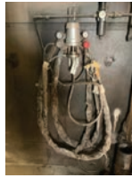
135 Finish pump/ with kremlin spray gun (paint use)
