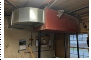
142 Air make up system / Powermatic model GA-115/518,000 BTU-230 volt
