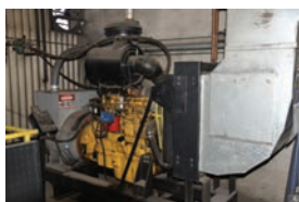
LOT 301 JD Engine Set up with Generator Engine Model # 6081AF001|Serial # RG6081A110858|HRS 31,415|270 HP|Generator Mounted on Engine|Marathon -Lima Mac|3phase 480volt|175KW
